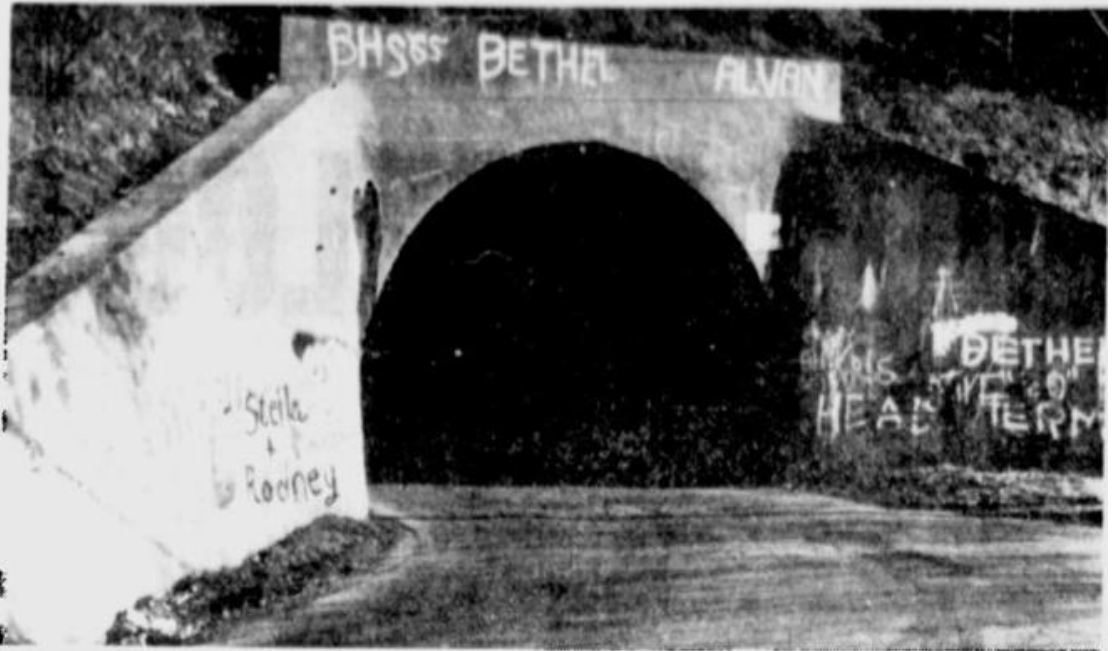
This is how Logan Road tunnel in Bethel Park looked after years of painting pranks.
