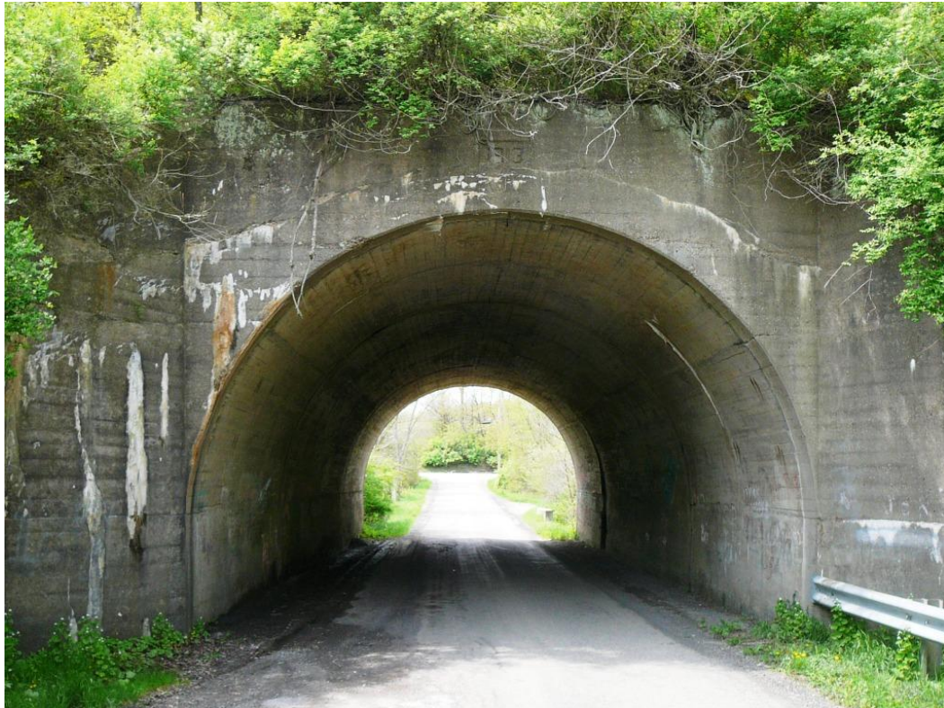
Looking west - 1913 in concrete on east side of arch
