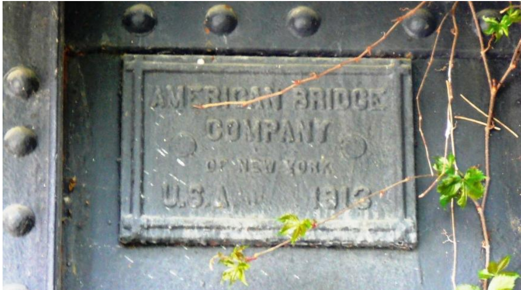
Builder's Plate – American Bridge Co. of New York U.S.A. 1913
