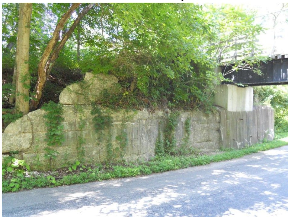
Additional concrete abutments on the south side indicate where a second span was located that led into the National # 2 Mine yard tracks.
