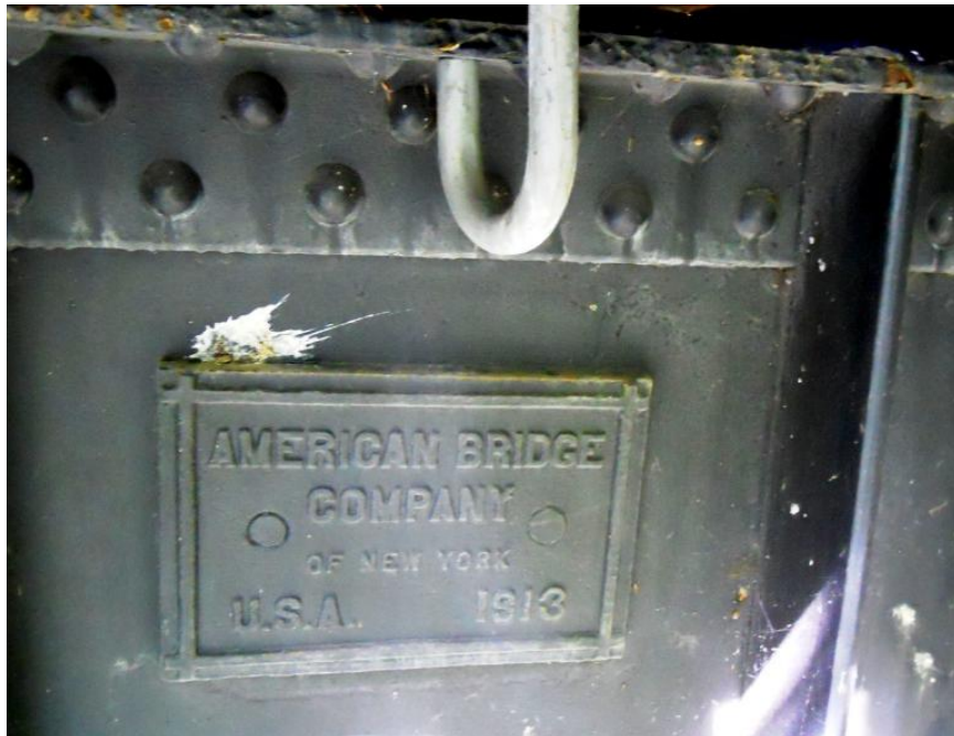
Builder's Plate – American Bridge Co. - dated 1913
