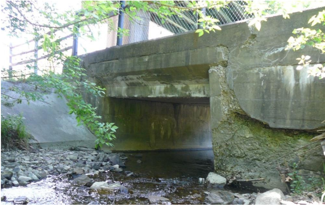
Looking west with Beaver Grade Road overpass in background
