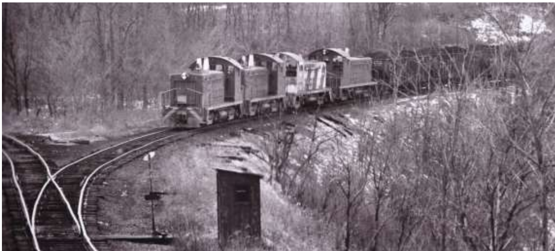
A railroad telephone booth sits beside the west switch at North Star Junction.
