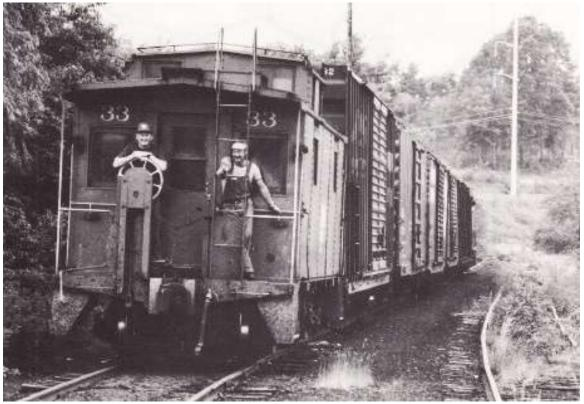
A train from Brookside Lumber backs through the east leg of the wye track. It will then pull out on the west leg of the wye with the locomotive leading the train. The storage siding can be seen to the right of the train. Gene P. Schaeffer photo.
