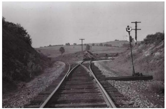
Looking east at the west wye switch. The main line to Bethel Park curves to the left and the west leg of the wye diverges to the right. Loaded hoppers can be seen sitting on the storage siding along the east leg of the wye in the background. Photo from Gene P. Schaeffer collection.
