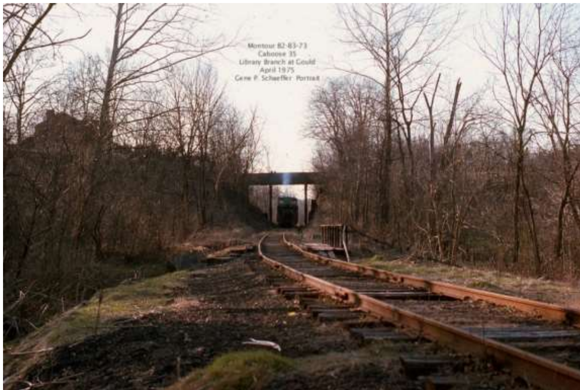
A train shoves under Triphammer Road. After abandonment of the railroad, the bridge was removed and the cut filled in. The current trail runs to the left of the tracks. Gene P. Schaeffer photo.
