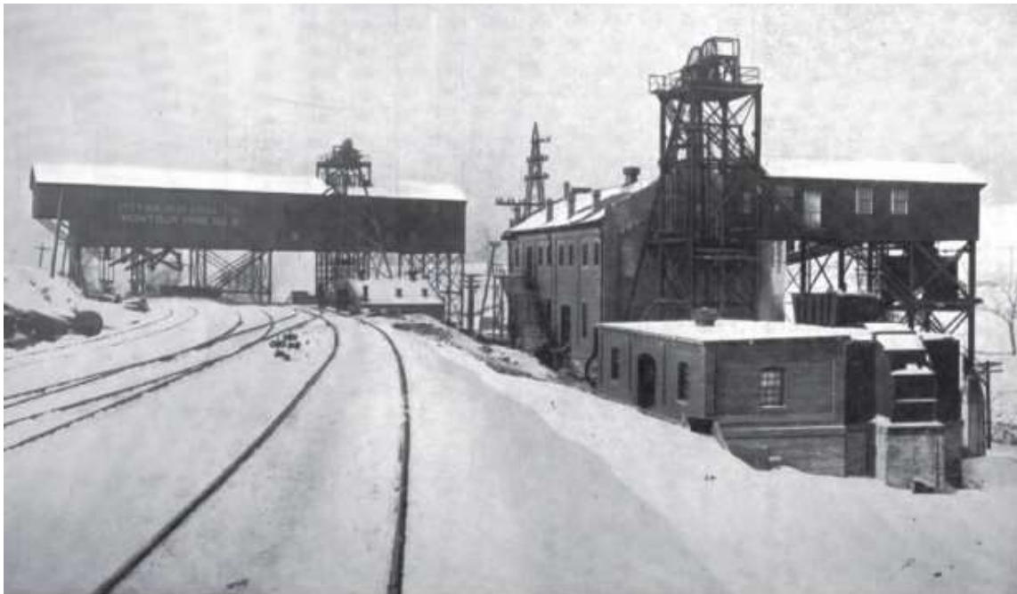
Montour #2 was a shaft mine, with support buildings next to the shaft in the foreground and the tibble building with its hoist shaft in the background. Photo courtesy Gene P. Schaeffer collection.
