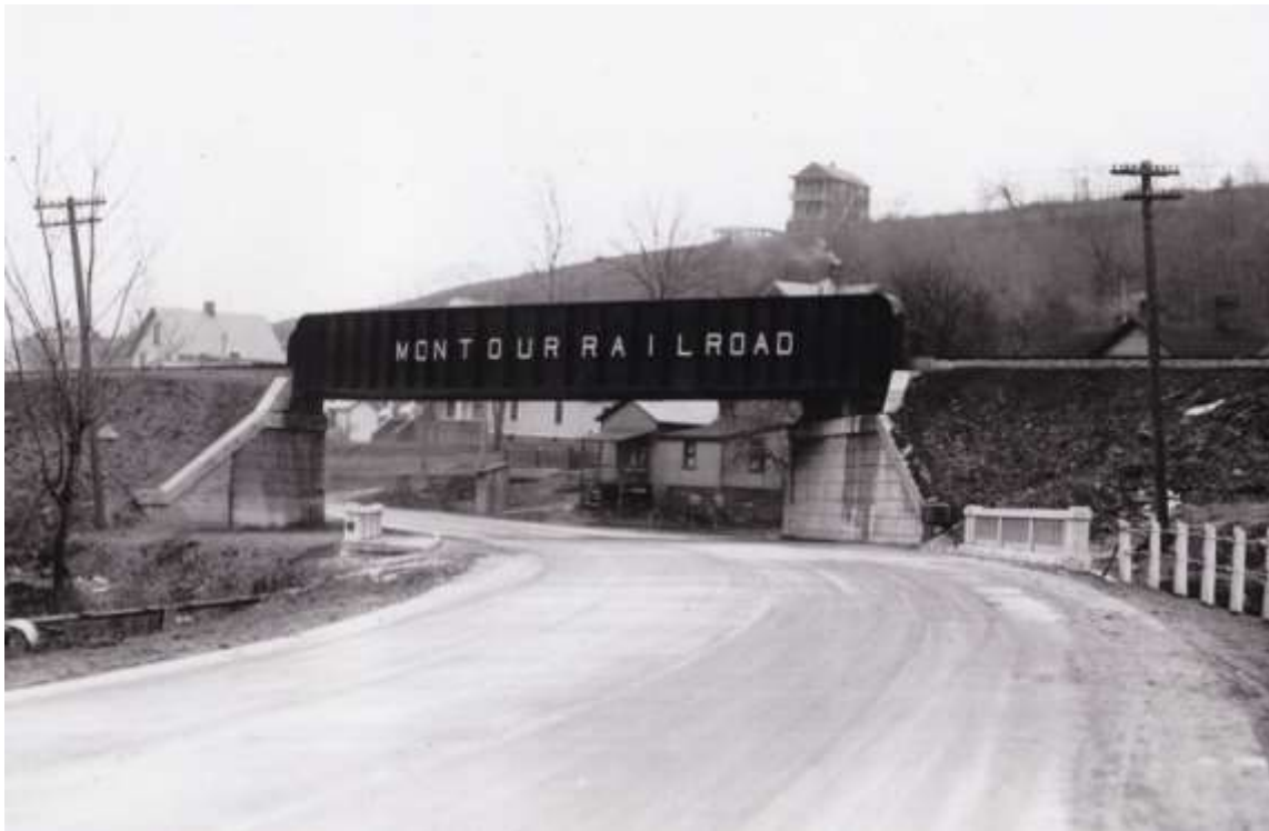
A 1930 view of the then new bridge over Route 30 in Imperial, which eliminated a grade crossing. County of Allegheny photo from Gene P. Schaeffer collection.
