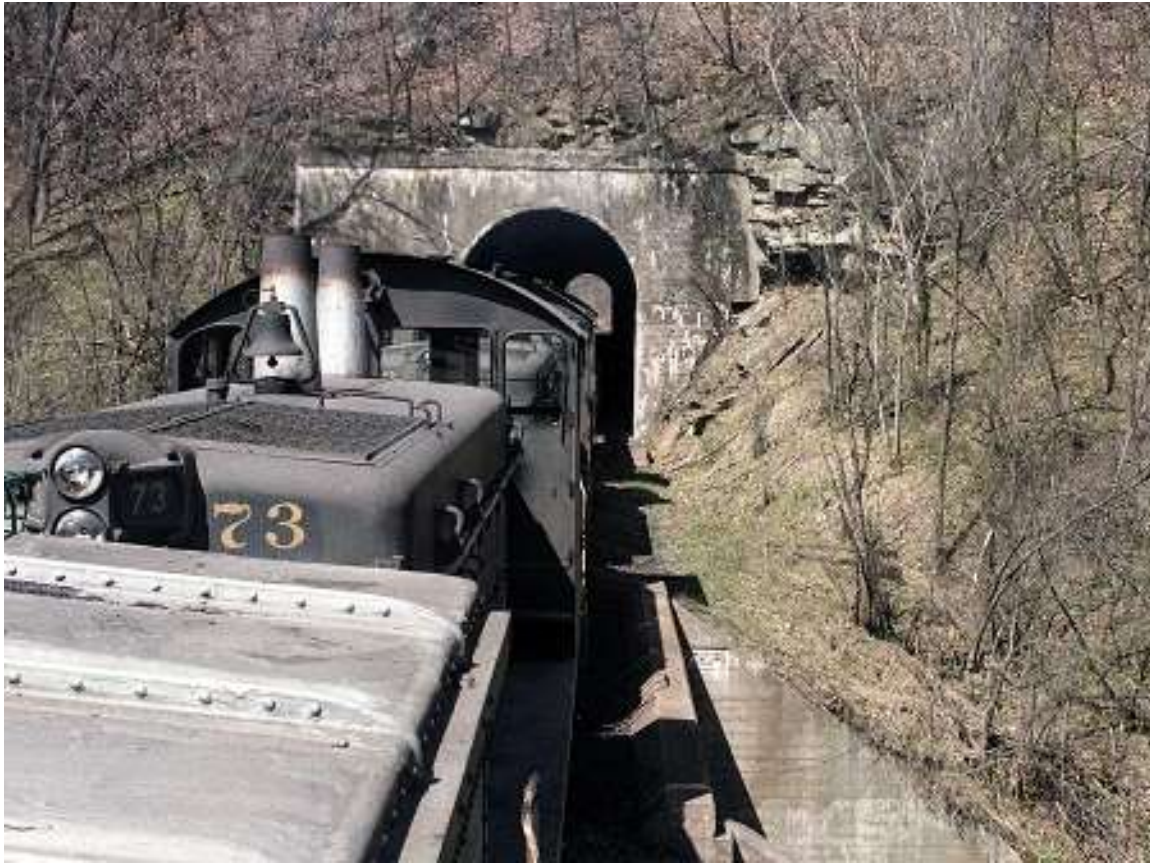
A view from a caboose shows a train crossing the concrete slab bridge before entering Enlow tunnel. A date stamp can be seen in the concrete bridge abutment. Roy E. Parkinson photo from Gene P. Schaeffer collection.
