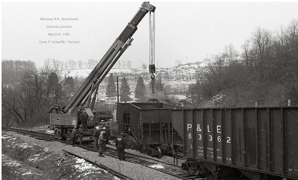
Empty hoppers headed to Westland derail at the Gilmore Junction switch, March 1981. A truck crane has been called in to re-rail the cars. Gene P. Schaeffer photo.
