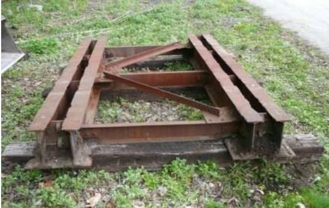
Lotus bridge relocated to Mile 30. The main I-beams and cross bracing are evident in this view without deck ties and rails. Bryan Seip photo
