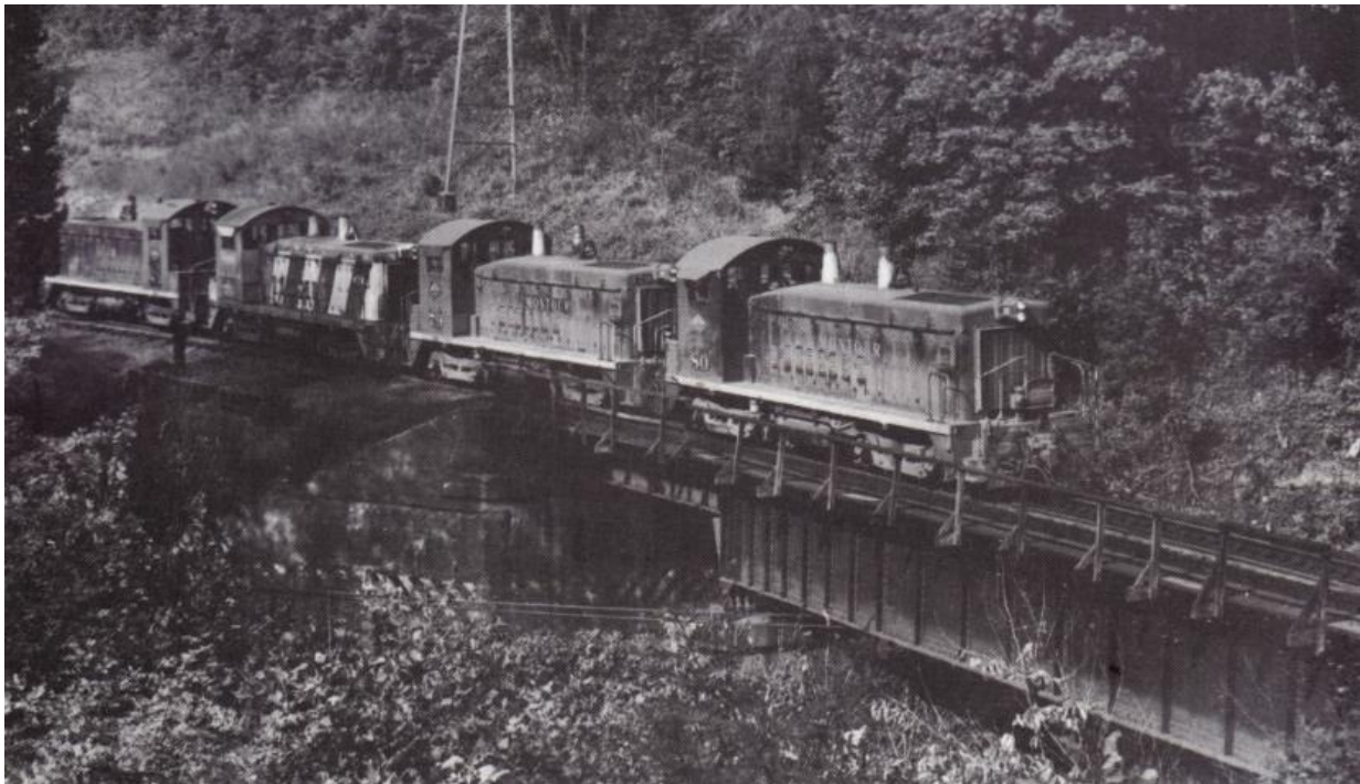
Four diesel locomotives lead a train eastbound across the bridge in 1979. Gene P. Schaeffer photo
