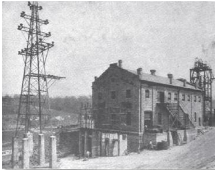
FIG. 3. REAR VIEW OF SUBSTATION AT MONTOUR MINE NO. 2
