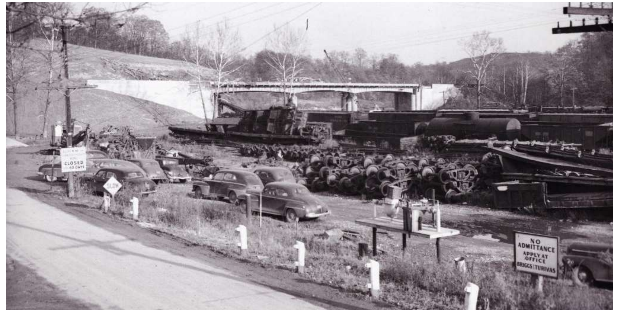
The Briggs & Turivas yard is filled with rail cars and recovered parts in 1948. In the background, construction is taking place on the Parkway West. Allegheny County Department of Public Works archives photo.
