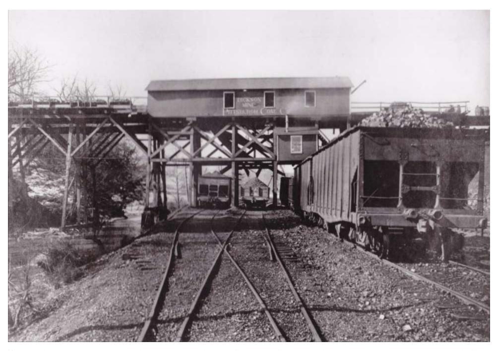
Seen in 1915, the Dickson Mine tipple sits beside Montour Run. After cleaning and sorting, mined coal was loaded into railroad cars. Pennsylvania State Archives photo courtesy Gene P. Schaeffer.
