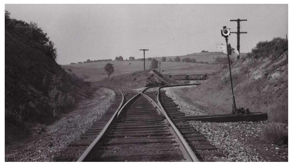
This 1944 view shows the west switch of the junction set for the main line curving to the left toward Bethel Park. The diverging track to the right continued toward Library. Loaded coal hoppers can be seen in the background, stored on the siding along the east leg of the wye.
